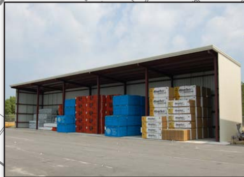
3-Sided Bulk Shed
