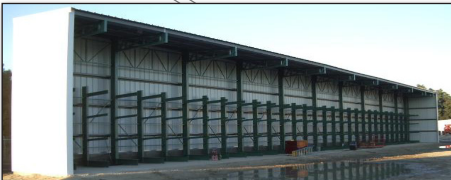
L-Shed with End walls
