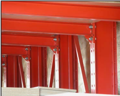
Structural Steel Racking
