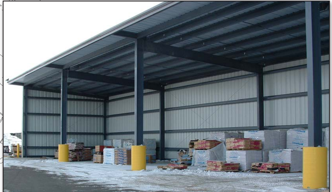
Bulk Shed with Column Protectors
