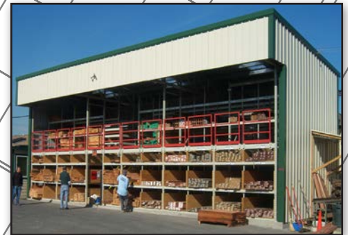
Shed with Board Rack Mezzanine
