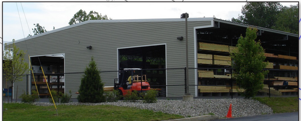
Drive-thru with Hardy Plank Siding
