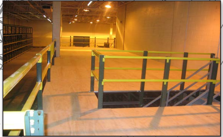
Mezzanine above bin storage
