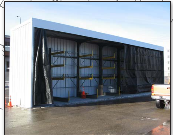
L-Shed with Shade-Dri Protection
