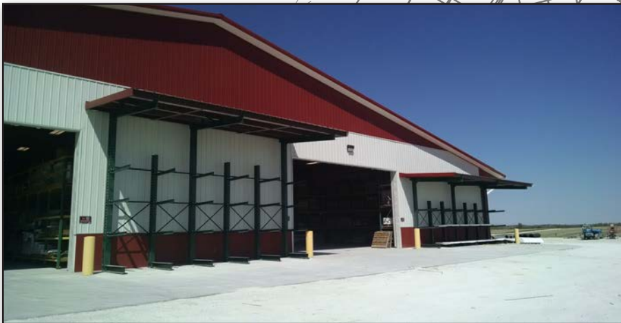
L-Sheds against Existing Building
